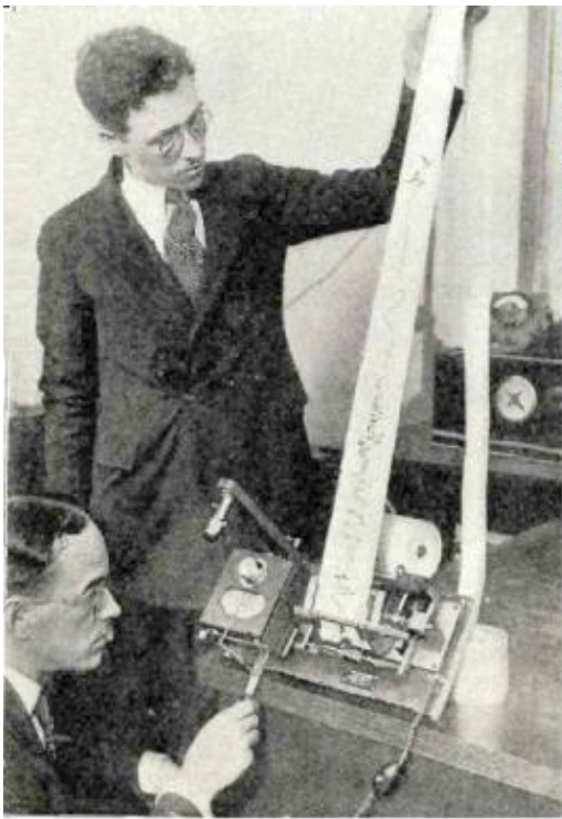
L: Apparatus used by engineers at the RCA laboratory in New York City to record signal level variations during the 1925 eclipse.
